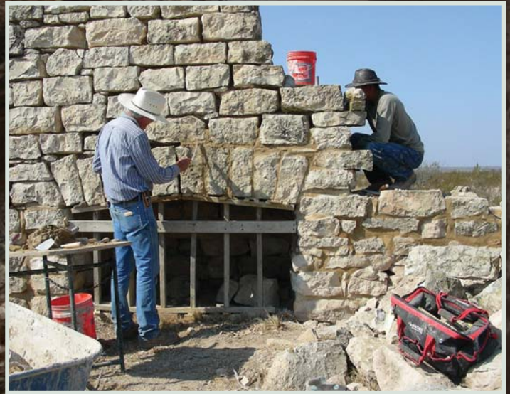
Stabilizing structural remains at Camp Meyers.
